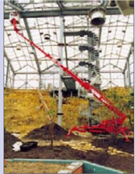
Assembling glass elements
